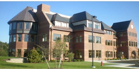
NORTH EASTON SAVINGS BANK Easton, MA 30,500 SF Collaboratively w/FCI
