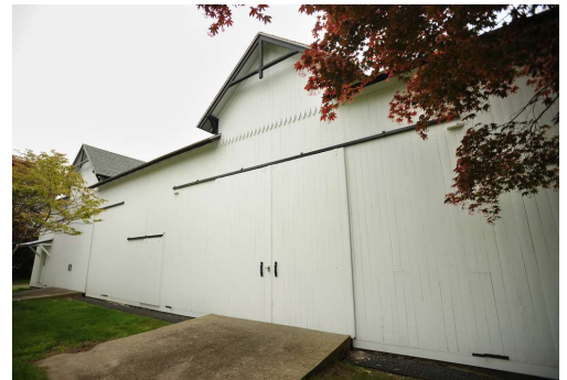
▲ Stowe Barn (c. 1851) Milford, CT
