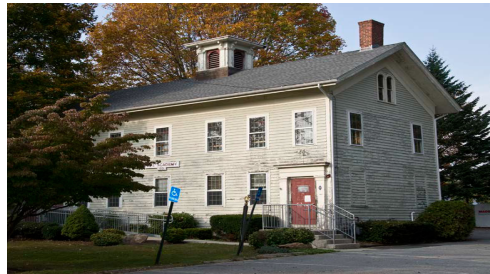
▲ Academy Building (c. 1801) Clinton, CT
