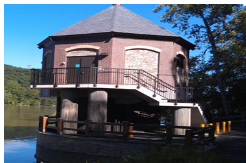
▲ Kleen Energy Pump Systems & Housing Middletown, CT (Power Generation)
