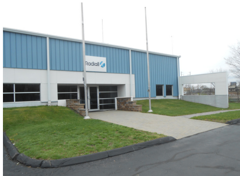
▲ Radiall Corporation Consolidation New Haven, CT (Connectors and Components)
