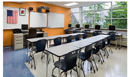
▲ Classroom renovation, Alternative High School, Waterbury
