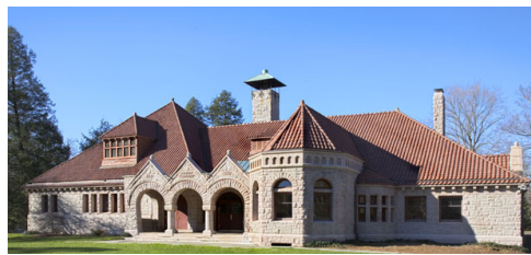
▲ Pequot Library (c. 1889), Southport, CT M/E/P Engineering Design Services
