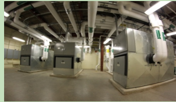
132 vertical bores and earth loop headers (left) comprise the geothermal system (center) @ Chatfield-LoPresti School in Seymour and ceiling mounted active chilled beam technology @ Berlin High School (right).
