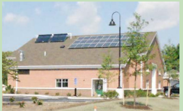
Solar photovoltaic panels for electricity and hot water @ Fire House #5 in East Hartford, a LEED™ Gold facility.
