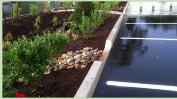
Rainwater harvesting for re-use and vehicle washing @ Fire Headquarters in Branford.
