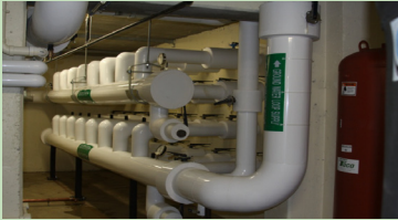
132 vertical bores and earth loop headers (left) comprise the geothermal system (center) @ Chatfield-LoPresti School in Seymour and ceiling mounted active chilled beam technology @ Berlin High School (right).
