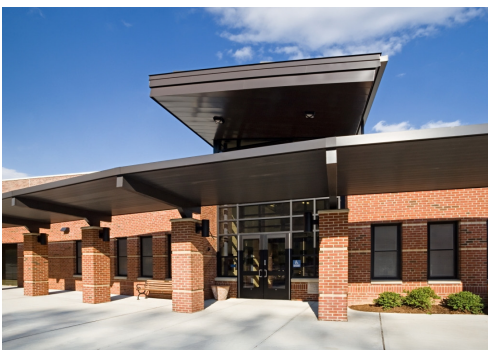
Stratfield Elementary School ♦ Fairfield, CT 513 students 58,000 SF $15,300,000
